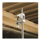
• Conforms with Federal Specification WW-H-171 (Type 23), Manufacturers Standardization Society ANSI®/MSS-SP-58 (Type 19 and 23)
